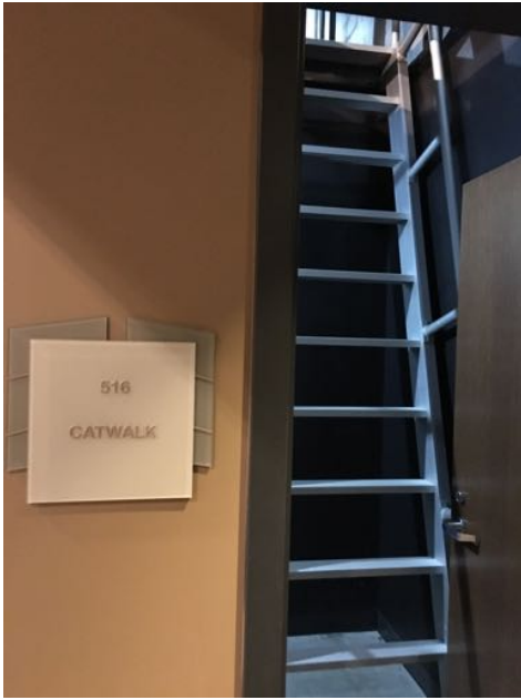
Stairway to catwalk
